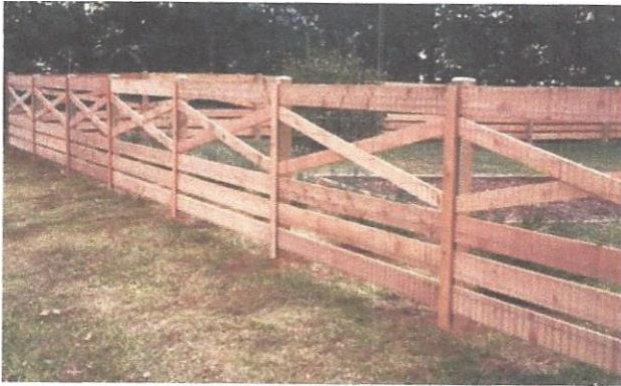
Six Board Estate Fence
